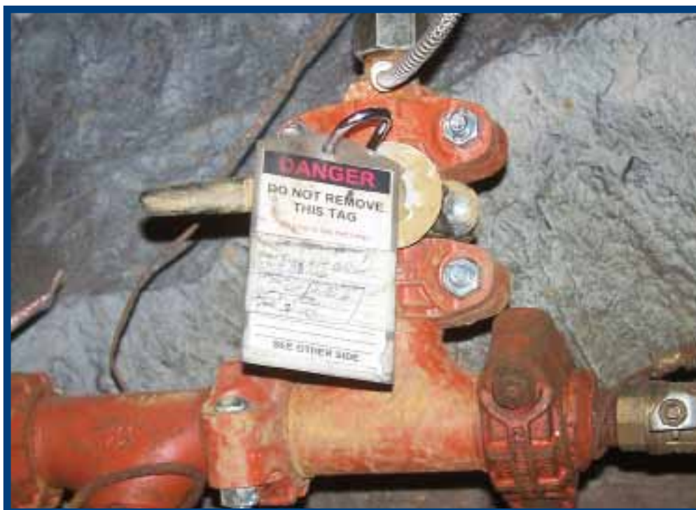
Victaulic valve lockout system. Equipment should be TSSA approved and have a Canadian Registration Number (CRN) which complies with standards set out by Canadian Standards Association (CSA). Picture courtesy of Victaulic.
