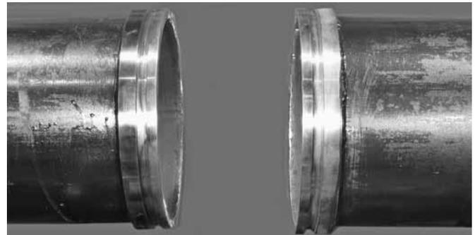
2. Support both sides of the pipe securely. Allow enough clearance to pass the coupling housing between the two pipe ends. **NOTE:** Pipe support must be maintained throughout the entire installation procedure, until instructed otherwise.
