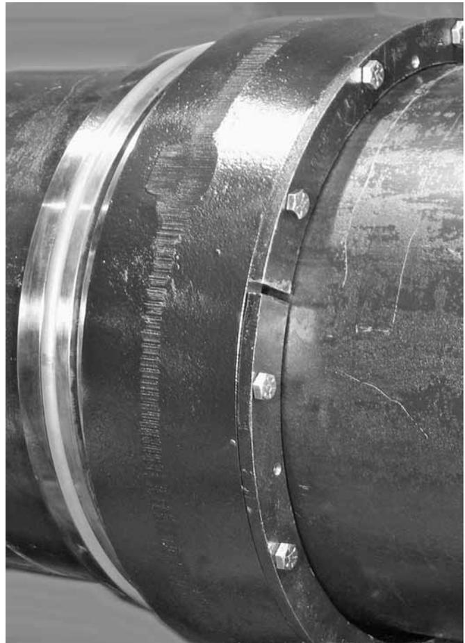
7. On the side of the coupling housing away from the Vic-Rings, install two end-retainer half rings. Make sure the markings on the end-retainer half rings are facing out. Thread 1/2 - 13 x 1 1/2-inch long Grade 8 hex-head cap screws through each outside hole in the end-retainer half rings and into the coupling housing, as shown above. Tighten the hex-head cap screws completely.
