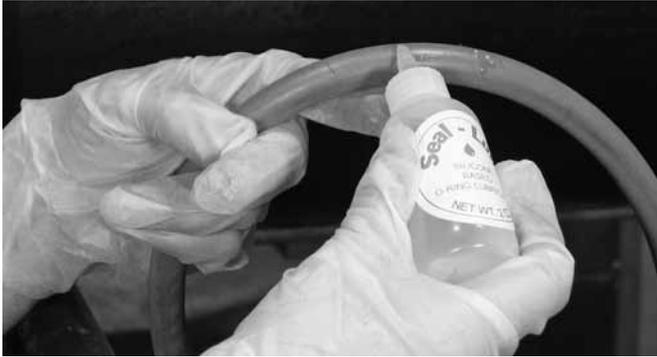
4. Lubricate the o-rings thoroughly with Seal-Lube™ O-Ring Lubricant\* supplied by Victaulic. Prevent dirt and debris from contacting lubricated o-rings.
