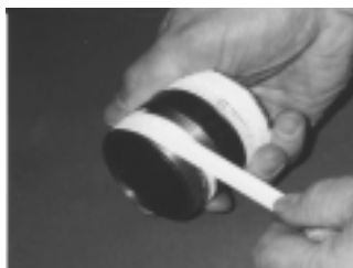
Step 2: Apply suitable pipe dope or teflon tape to the 2" (50 mm) nipple (Item #4).
