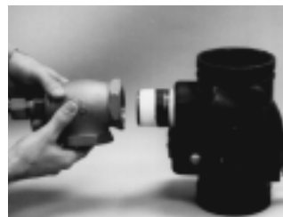
Step 11: Install the 2" (50 mm) 90° angle valve (Item #1).
