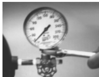
Step 7: Install the water pressure gauge (Item #3).
