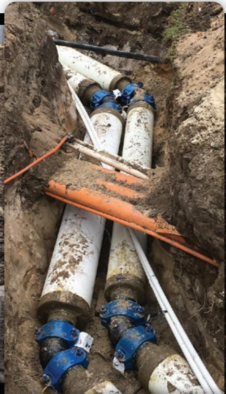
*Victaulic* Style 905 couplings were selected by this university for their plain-end installation method. Pipes were laid pre-insulated and easily joined together directly in the trench, making the process extremely simple and efficient.
