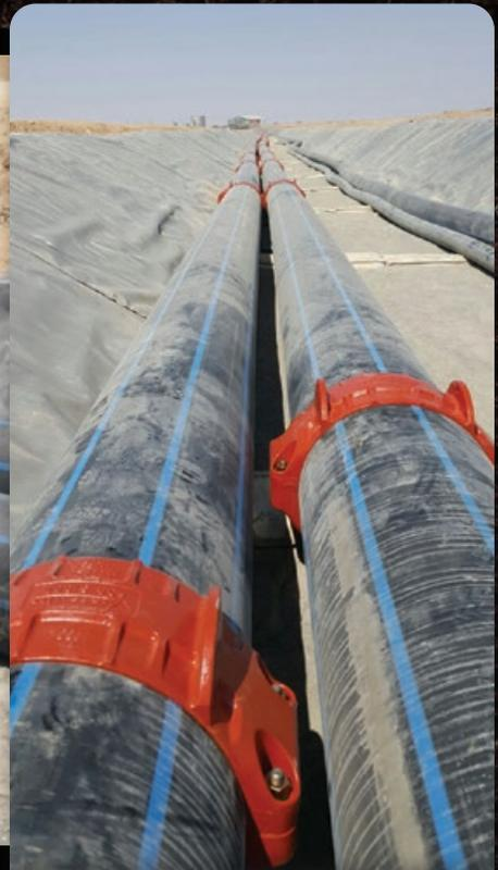
When considering a pipe joining method for their 2.5 mile | 4 kilometer long, 24" | 630 mm OD HDPE tailings pipeline at Husab Uranium Mine, the Husab Joint Venture sought a solution that would allow for ease of future maintenance and a fast initial installation.
