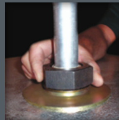
Tighten hex nut by hand and 3/4 turn of a wrench
