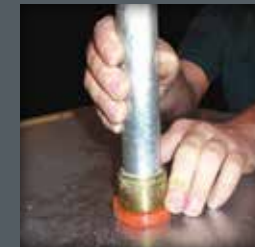
Slide rubber seal, backing plate, lock washer, and hex nut down V36 Sprinkler
